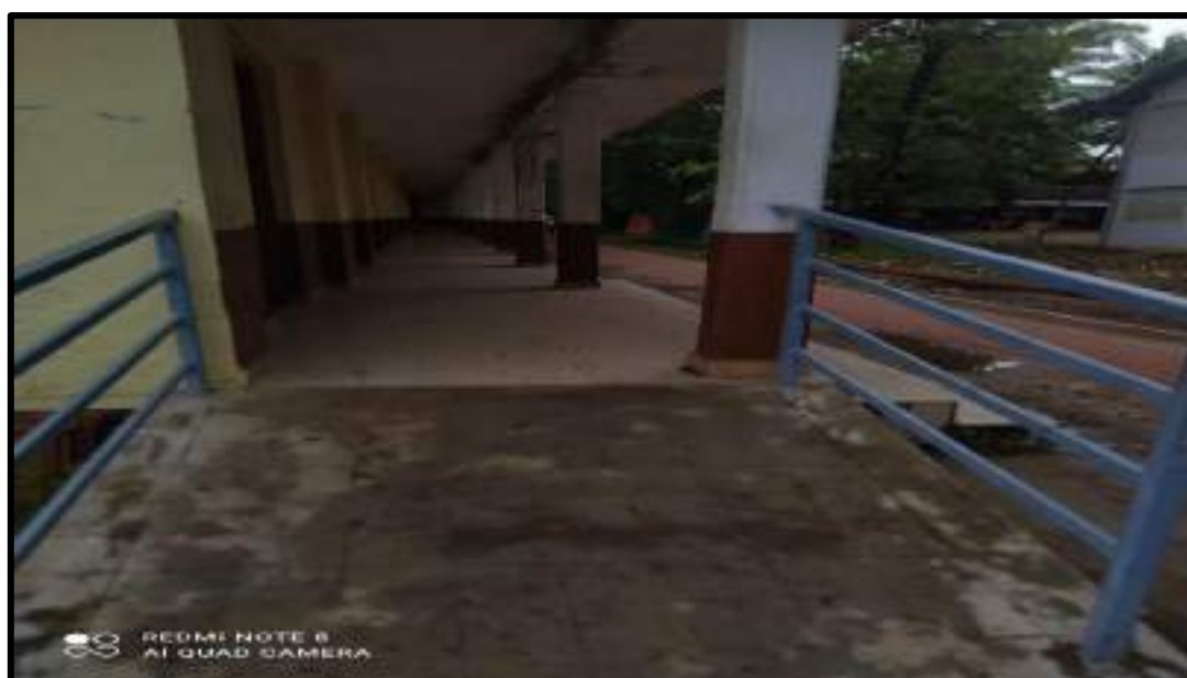
Ramp at Old Block
