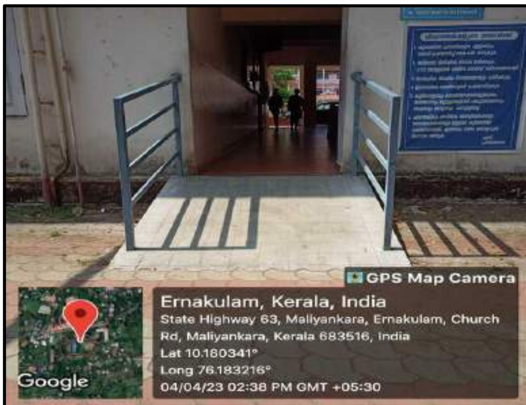
Ramp at Main Block
