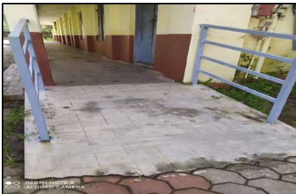
Ramp at WS Block
