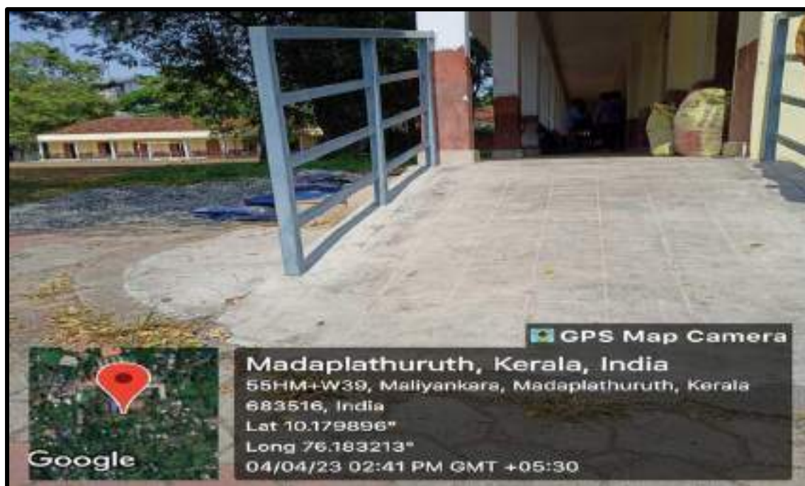
Ramp at Old Block
